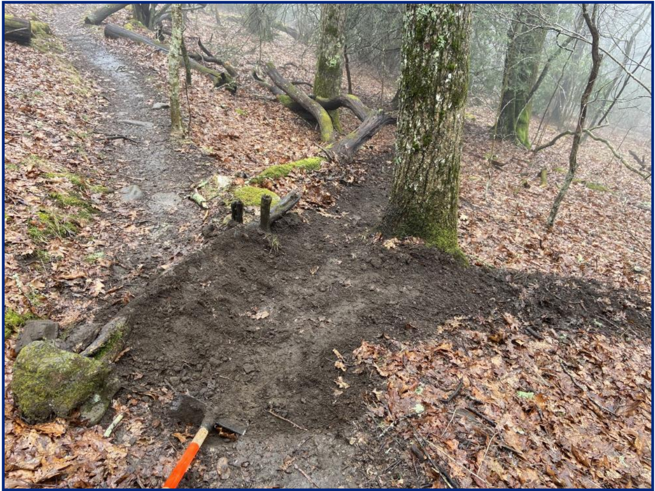
A recently maintained water bar, submitted by Bill Van Horn
