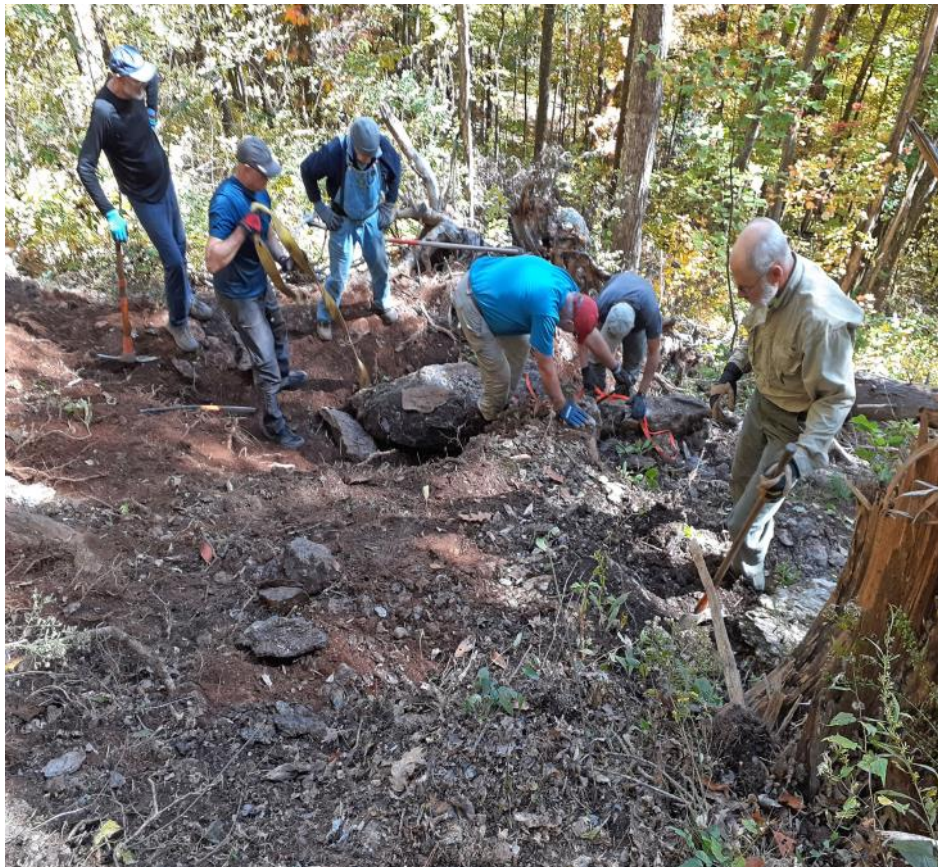
Positioning rock after it was moved into the hole to support the new treadway.
